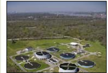
Sewage Treatment Facility in Gretna (Jefferson Parish), Louisiana (David R. Frazier Photolibrary, Inc./Alamy.)
